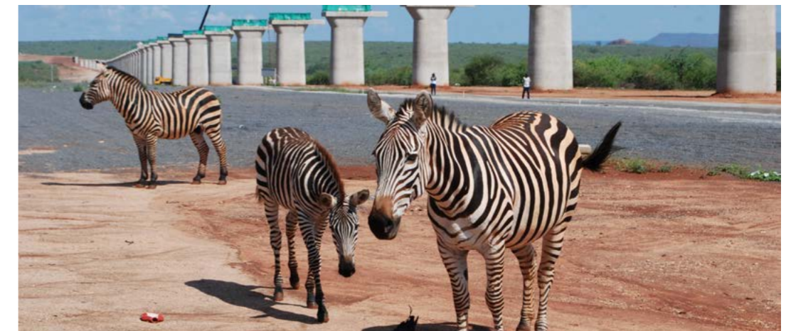
中国路桥在蒙内铁路沿线设置野生动物通道 China Road & Bridge Corporation set up wildlife passageways along Mombasa-Nairobi Railway.
