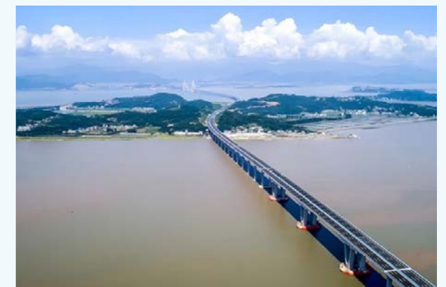
一公局集团：一种变截面节段梁短线预制拼装方法（乐清湾大桥） CCCC First Highway Engineering Group: A Short-line Prefabricated Assembly Method of Variable Cross-section Segment Beams (Yueqing Bay Bridge)
