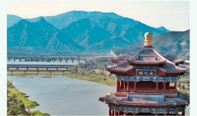
永定河流域综合治理与生态修复项目 Yongding River Basin Comprehensive Management and Ecological Restoration Project
