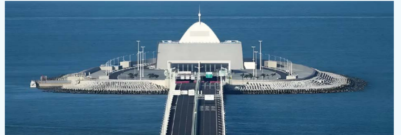
中国交建承建的港珠澳大桥主体工程岛隧工程 Island tunnel engineering, the main works of Hong Kong-Zhuhai-Macao Bridge, undertaken by China Communications Construction
