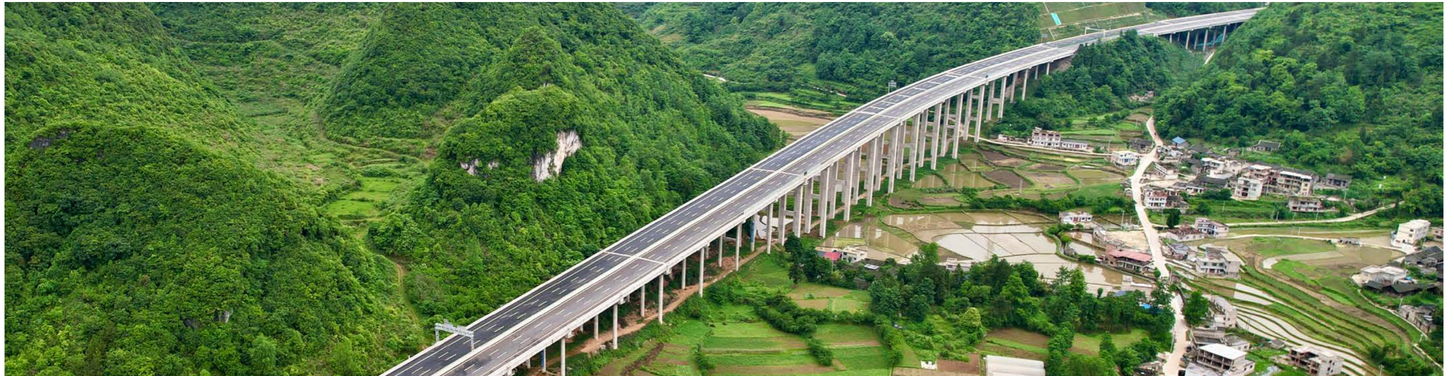
广连高速三凤里互通至连州段 Sanfengli Interchange to Lianzhou Section of Guangzhou-Lianzhou Expressway
