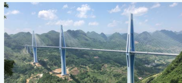
二公局承建的平塘特大桥 Pingtang Bridge undertaken by CCCC Second Highway Engineering Co., Ltd.
