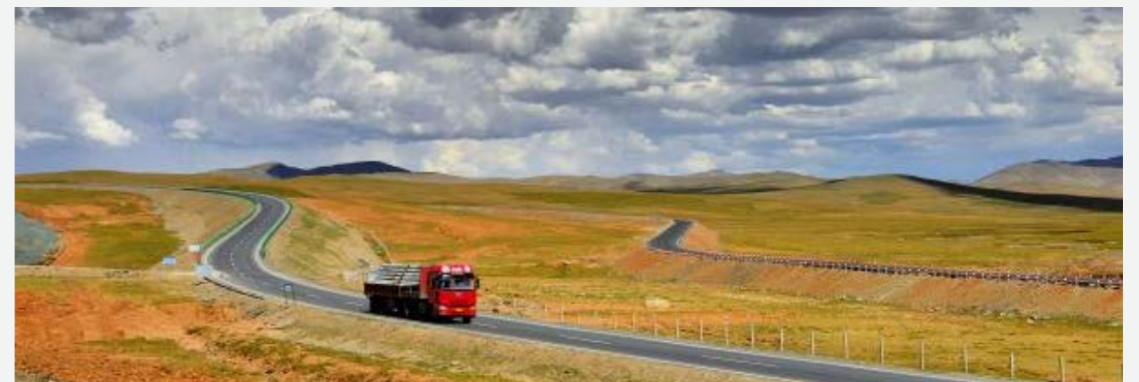
中国交建支撑建成世界首条高海拔高寒多年冻土区高等级公路——共玉高速公路 The First High-grade Expressway at High Altitude and the High Code Area and Permafrost Region Supported by China Communications Construction in the World —Gonghe - Yushu Expressway
