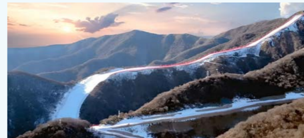
一局集团承建的国家高山滑雪中心项目 National Alpine Skiing Center Project undertaken by CCCC First Highway Engineering Group Co., Ltd.
