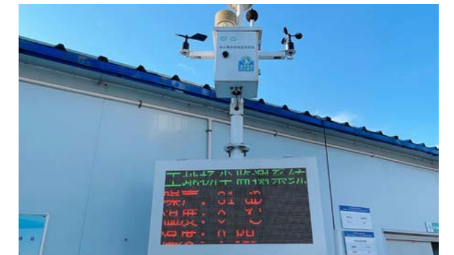
工地扬尘监控系统 Dust monitoring system on construction site
