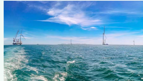
国内首个成规模单机容量 5 兆瓦直驱型风机的海上风电场——中闽福建平海湾海上风电场 First large-scale offshore wind farm in China with a single unit capacity of 5 MW with direct-drive fan - Zhongmin Fujian Pinghai Bay Offshore Wind Farm
