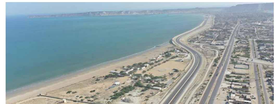
中国交建承建的巴基斯坦瓜达尔港东湾快速路项目通车 The Dongwan Expressway Project in Gwadar Port, Pakistan, undertaken by China Communications Construction, was opened to traffic
