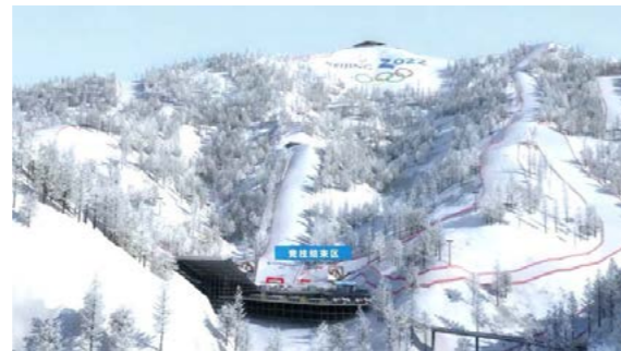
一公局集团承建国家高山滑雪中心第二标段 The construction of the second bid section of the National Alpine Skiing Center is undertaken by CCCC First Highway Engineering Group Co., Ltd.
