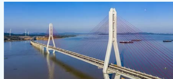
中国路桥承建的都昌至九江高速公路鄱阳湖二桥 The Second Poyang Lake Bridge of Duchang-Jiujiang Expressway undertaken by China Road & Bridge Corporation
